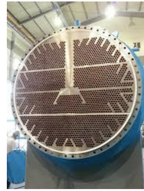
Gambar 1. Surface Condenser PLTU
